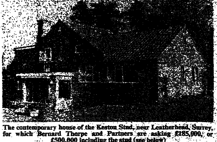
The contemporary house of the Keston Stud, near Leatherhead, Surrey, for which Bernard Thorpe and Partners are asking £185,000...
